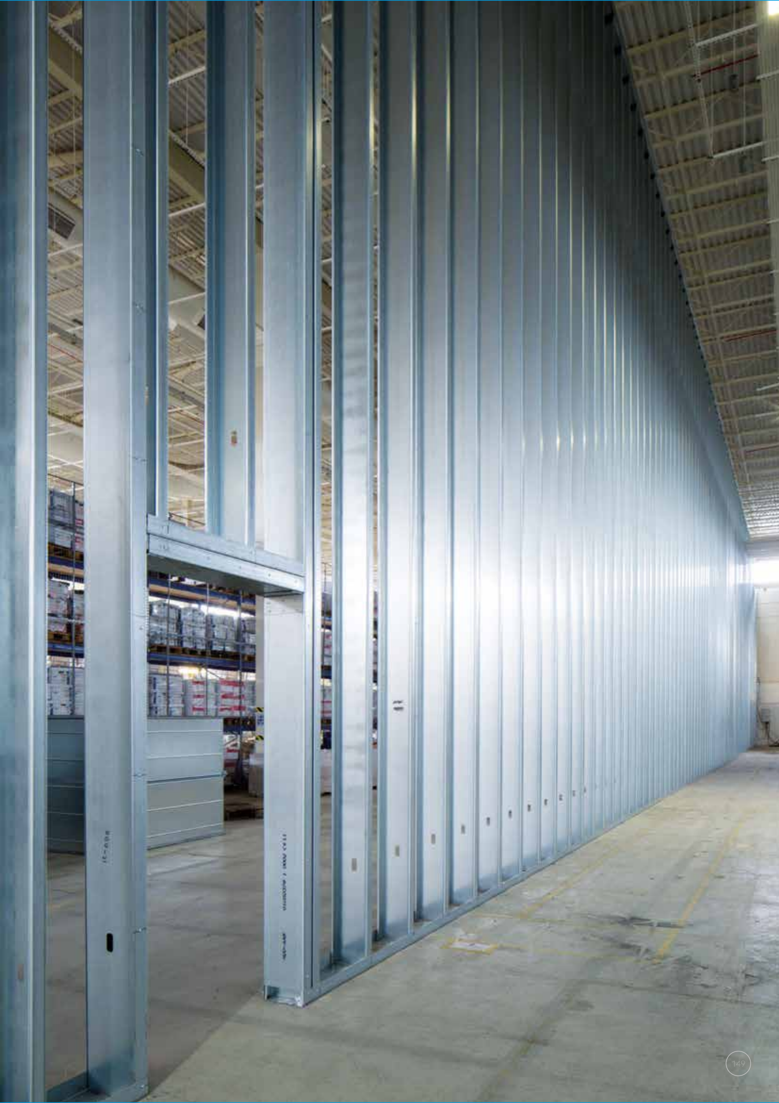
High Bay Walling
